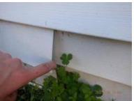
[CR] The manufactured siding was damaged/deteriorated at a lower area of the building by the attached workshop. These conditions are conducive to moisture intrusion/deterioration. We recommend correcting the condition(s) noted.
