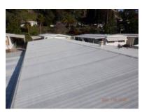
[CR] Some seams need to be re-sealed. These condition(s) are conducive to moisture intrusion and deterioration. We recommend correcting the condition(s) noted.
