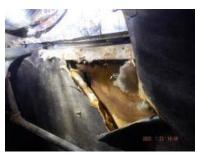
[CR] The rodent barrier was damaged/missing in areas. We recommend correcting the condition(s) noted.
