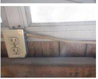
[SC] There was improper wiring installed in the form of extension cords or cord-type wiring. This type of wire is for temporary use only. We recommend correcting the condition(s) noted.
