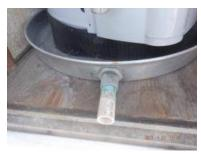
[CR] There was moisture staining and damage visible in the water heater cabinet. The area tested dry at time of inspection. We recommend locating and correcting the source and any damaged materials.
