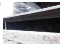
[CR] The gutters showed evidence of leakage at some seams. We recommend correcting the condition(s) noted.
