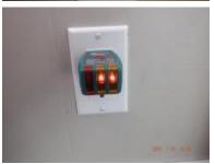
[NOTE] Hallway receptacle is GFCI protected and resets at the hallway bathroom.
