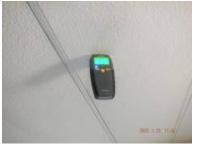
[CR] Moisture/stains were noted on the wall in the living room cabinet. The area tested dry during the inspection. We recommend locating and correcting the source as well as any damaged materials.
