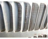
[CR] The coolant lines were not sealed to the wall were they entered the building. This condition allows for rodent access. We recommend correcting the condition(s) noted.
