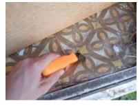
[CR] The insulation was installed in the wrong direction in the storage closet. We recommend correcting the condition(s) noted.
