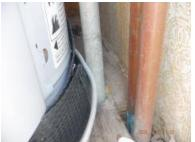
710 TANK: The water heater tank appeared serviceable, no leakage noted.
