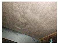
[CR] Water stains were noted in areas. The area was dry during the inspection. Monitoring the area for further staining and moisture evidence is recommended. If further moisture-related conditions are noted, corrective measures should be taken to eliminate the source of the moisture before deterioration results.
