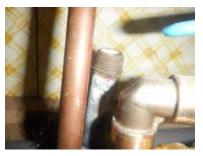
[NOTE] Galvanized steel pipes are outdated and subject to corrosion which will eventually result in restricted flow and leakage and will need to be replaced. Water flow in the home was satisfactory at the time of inspection.
