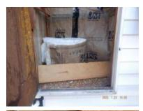
[FE] There was damaged wood on the door trim of the storage closet. We recommend further evaluation and corrections by a specialist in the appropriate trade.
