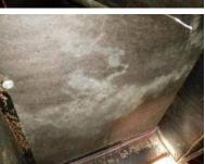
[FE] There was moisture staining and damage to the subflooring in some areas. The area tested dry at time of inspection. We recommend further evaluation and corrections by a specialist in the appropriate trade.
