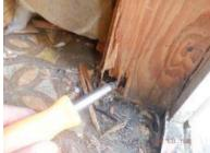
[CR] The workshop area showed evidence of moisture intrusion. We recommend locating and correcting the source and any damaged materials.
