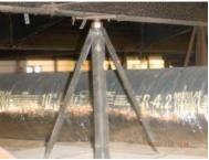
[CR] Some jack stands were rusted/deteriorated. We recommend correcting the condition(s) noted.
