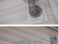
[SC] There was improper wiring installed in the form of nonmetallic sheathed wiring exposed to human contact and/or mechanical damage. We recommend correcting the condition(s) noted.
