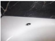
[SC] The hot and cold water were reversed at the faucet This condition is a scald hazard. We recommend correcting the condition(s) noted. [CR] The faucet(s)/spout were not sealed to the wall/deck. This condition is conducive to moisture intrusion into concealed spaces. We recommend correcting the condition(s) noted.
