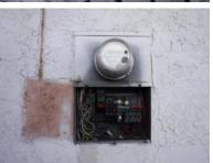
803 SERVICE RATING: 120/240 volt system, rated at 100 amperes.
