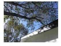
[CR] Tree(s) were planted too close to the building. We recommend considering removal, as trees continue to grow in size and damage may occur to the foundation, structure, plumbing system or roof. [NOTE] We recommend monitoring the conditions noted.
