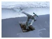
603 WATER PRESSRE: [FE] The water pressure was tested to be above 80 PSI, which exceeds the maximum per the building standards. See the "Water Pressure" comment below for the details.
