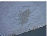
[RU] This building was built in an era before weep screeds were installed at the bottom edge of the stucco siding, the stucco was extended into the soil. The stucco wicks water up out of the soil which causes it to deteriorate from being moist for prolonged periods. We recommend minimizing moisture around the building to help protect the stucco and the foundation from moisture damage.
