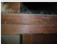
[FE] There was evidence of damaged wood framing in the attic. We recommend further evaluation and corrections by a specialist in the appropriate trade.
