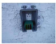
[SC] The GFCI receptacle at the right side of the building was providing power, but failed to trip when tested. This condition is safety hazard. We recommend correcting the condition(s) noted. [CR] One right side receptacle was mounted loose from the wall. We recommend correcting the condition(s) noted.
