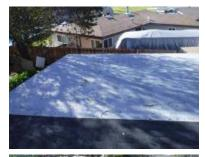
[CR] Evidence of ponding was noted. The presence of shallow ponds of water is not unusual. Regular maintenance of the areas is vital to prevent the build-up of vegetation, debris, sagging and possible damage to the roof.
