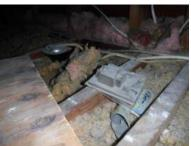
[CR] The flue was crushed and damaged. We recommend correcting the condition(s) noted.
