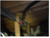
605 WASTE LINES: Materials: ABS black plastic piping and cast iron piping where visible.
